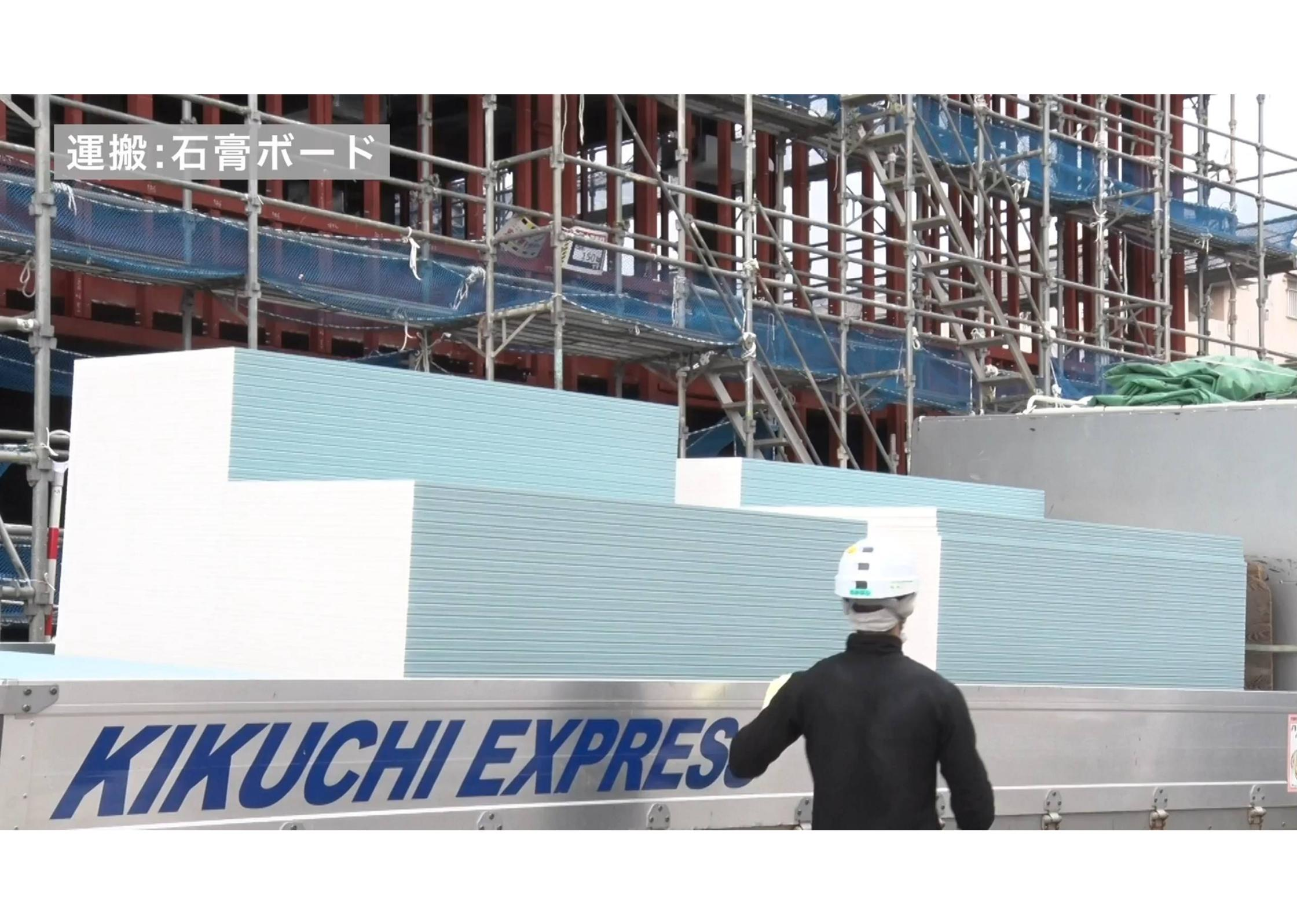
A construction worker wearing a white hard hat and a black jacket stands with his back to the camera, looking at a truck trailer. The trailer is loaded with several large stacks of gypsum board, some with white faces and others with blue faces. The truck is silver and has "KIKUCHI EXPRESS" written in blue on its side. In the background, there is a building under construction with extensive scaffolding and blue safety netting.
